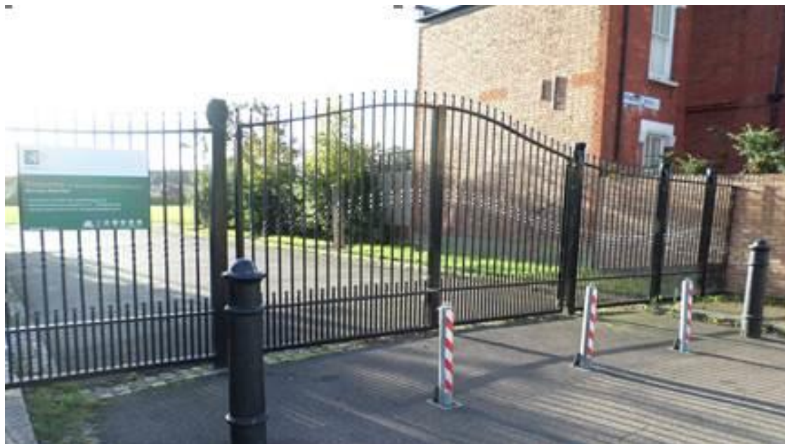
Image 21: Vehicle access gate at Boundary Road and within playground to Belmont School
