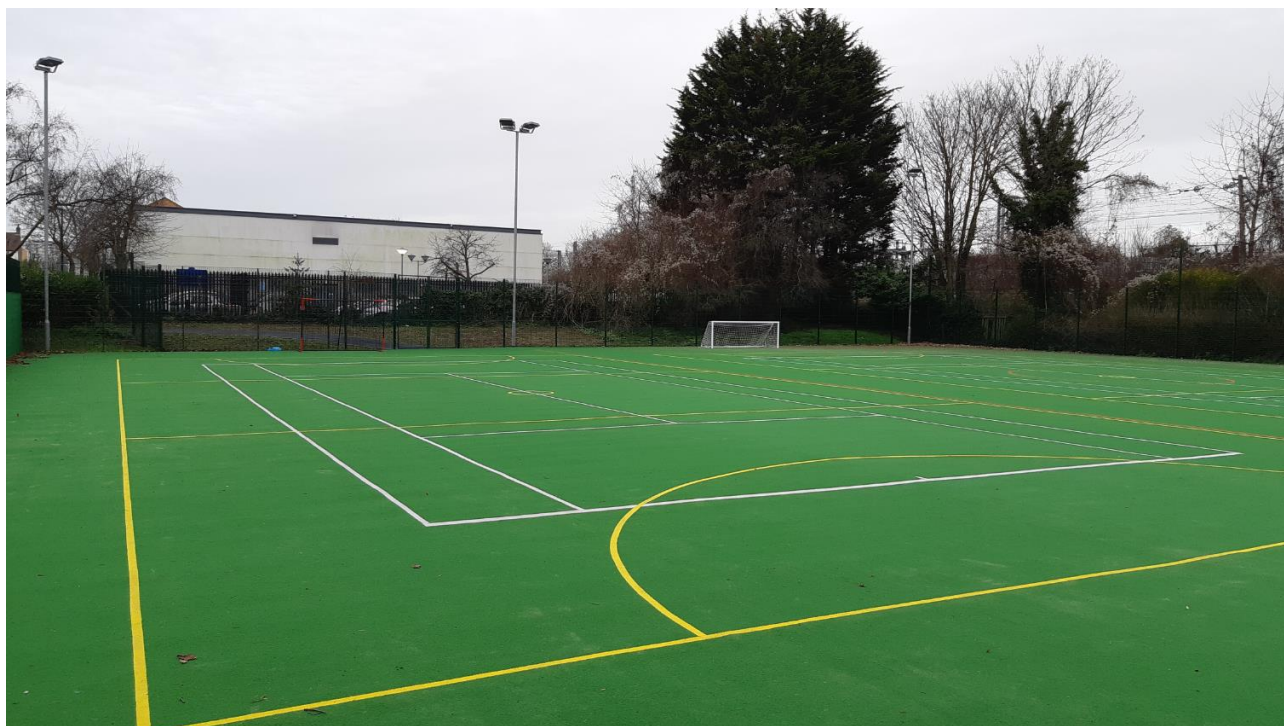
The new floodlit MUGA was completed in Autumn 2019
