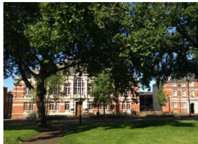
Civic green space of Tottenham Green with its mature trees flanked by impressive stand alone civic/educational buildings.
