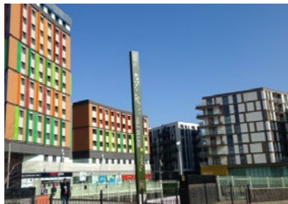
Recent, modern housing development comprising large, single blocks grouped around a network of public spaces
