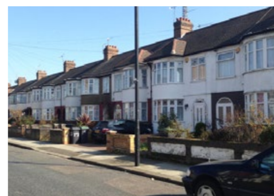
Interwar terraced houses just north along Shelbourne Road - wider and more horizontal than earlier Victorian houses with curved bay windows and larger setbacks from pavement which unfortunately has allowed people to pave over them for car parking.
