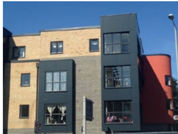
Modern apartment building with clever use of winter gardens to provide meaningful private amenity space on the busy Broad Lane.
