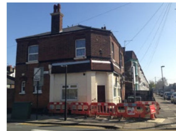
2 storey building with a chamfered edge - would have previously been a shop of some kind.
