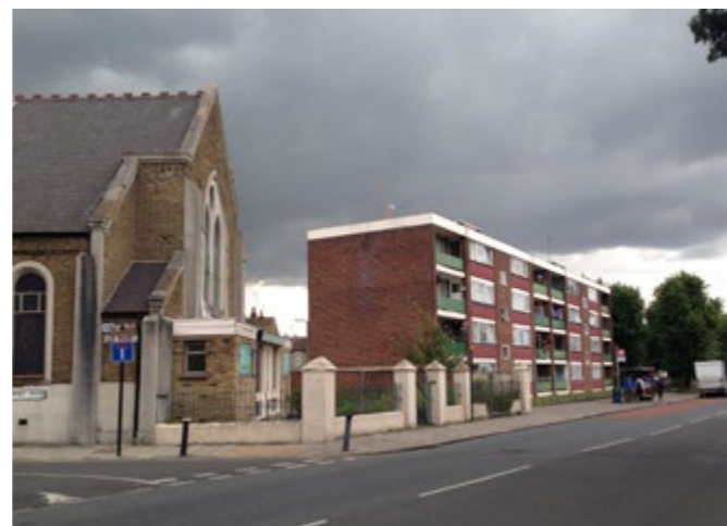
West Green Road - West Green Baptist Church next to an early postwar block of flats reflecting this important east-west streets mixed character and place of constant change.
