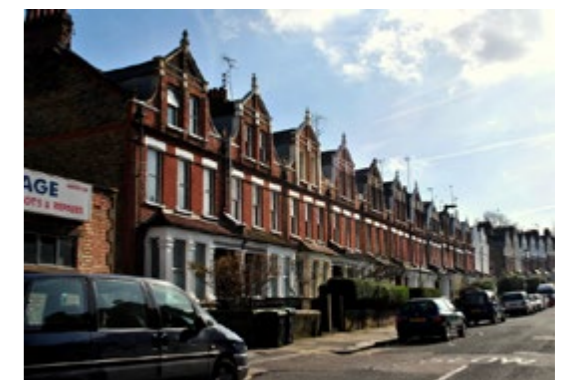
Rhythmic roof scapes and gentle topography adds interest to the otherwise homogenous terraces
