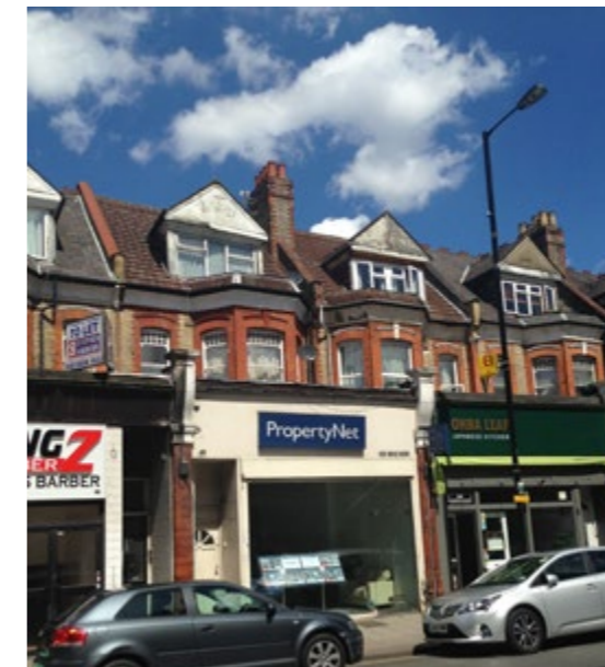
Nuclea centre - ground floor shopfronts with residential above
