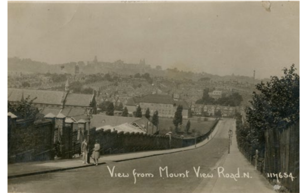
Mount View Road, looking north c1920-30
