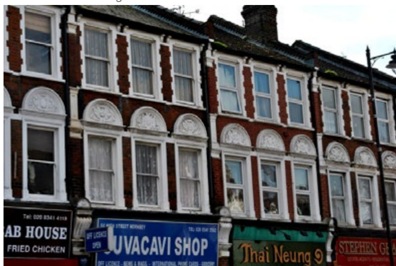
Decorative architectural details along Hornsey High Street, above retail parade
