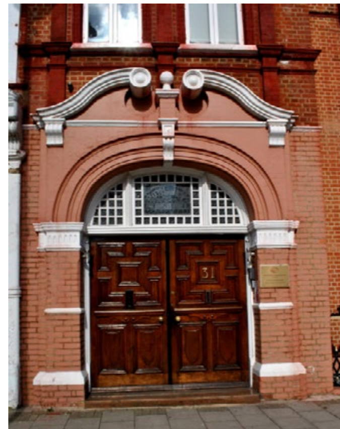
Entrance door to locally listed Community Centre, formally St Mary's Centre
