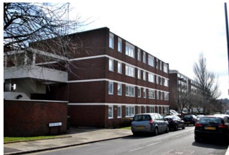
Estate blocks along Boyton Road
