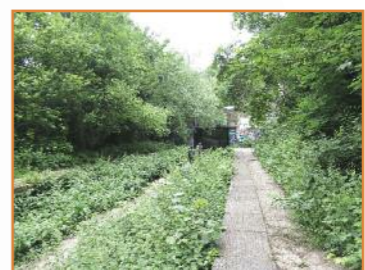
Remains of the station platform on parkland walk at Crouch Hill
