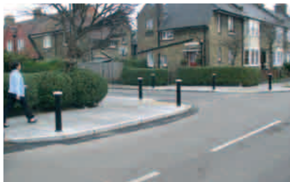
Kerb build-outs, Haringey
