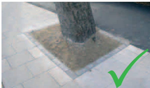
Good Practice - Porous Resin bound gravel tree pit, Wood Green
