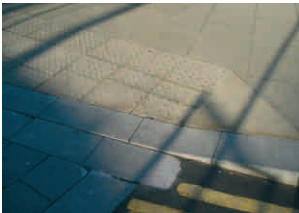
Tactile paving to match adjacent Yorkstone paving
