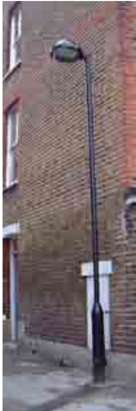
Haringey Standard - Residential Street, 5m. Flat glass is used to reduce light spill into adjoining properties.
