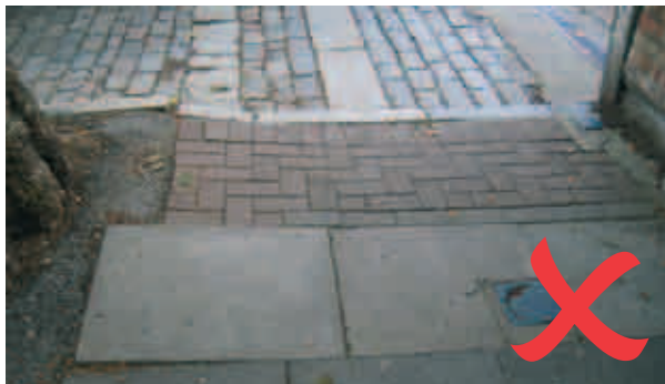
Bad practice - using different paving materials does not promote visual continuity
