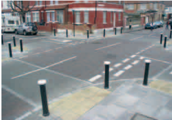
Junction treatment, Haringey
