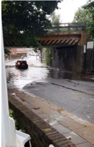
Figure 5-3 Flooding at Forster Road underpass, 25th July 2021
