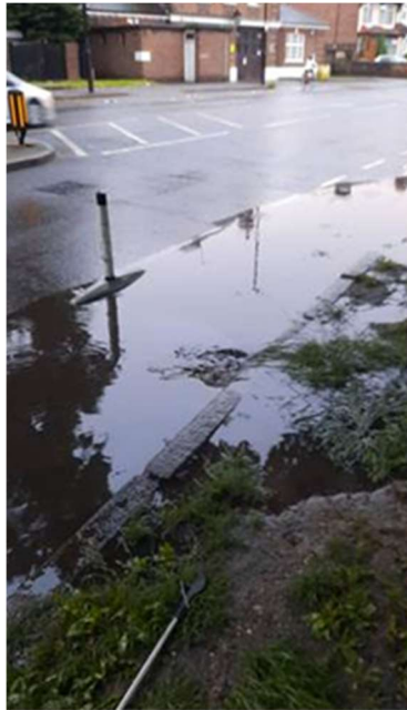
Figure 5-7 Flooding at Bounds Green Road (junct Nightingale Road), 12th July 2021
