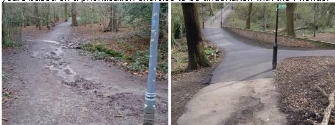
Image 13 & 14: Paths before and after the 2008/09 improvement works
