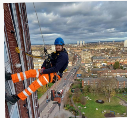
Specialist surveyor abseiling from the roof of Stellar House
