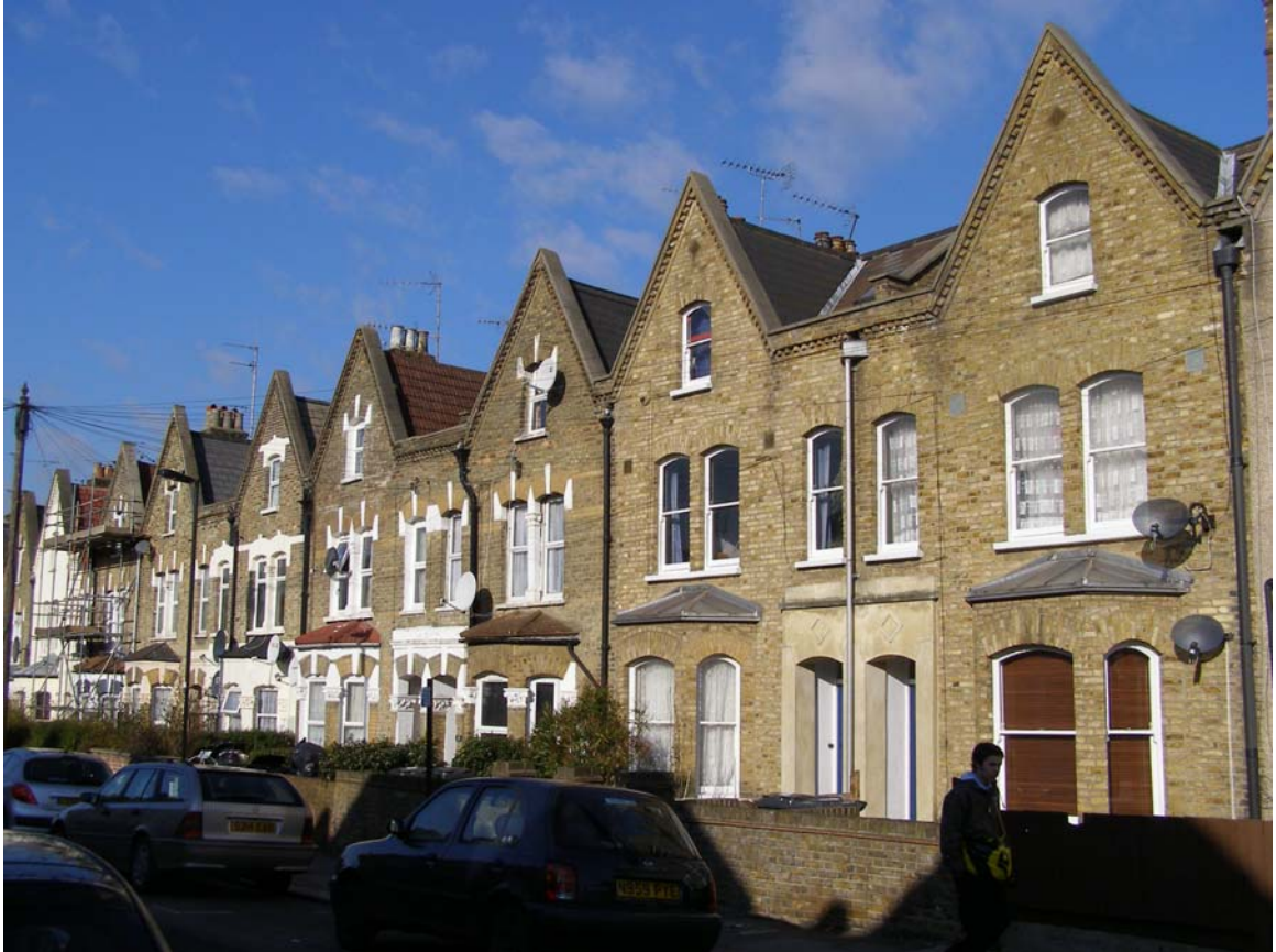
Figure 8; typical gable fronted terrace not suited to Type 2 and 3 extensions
