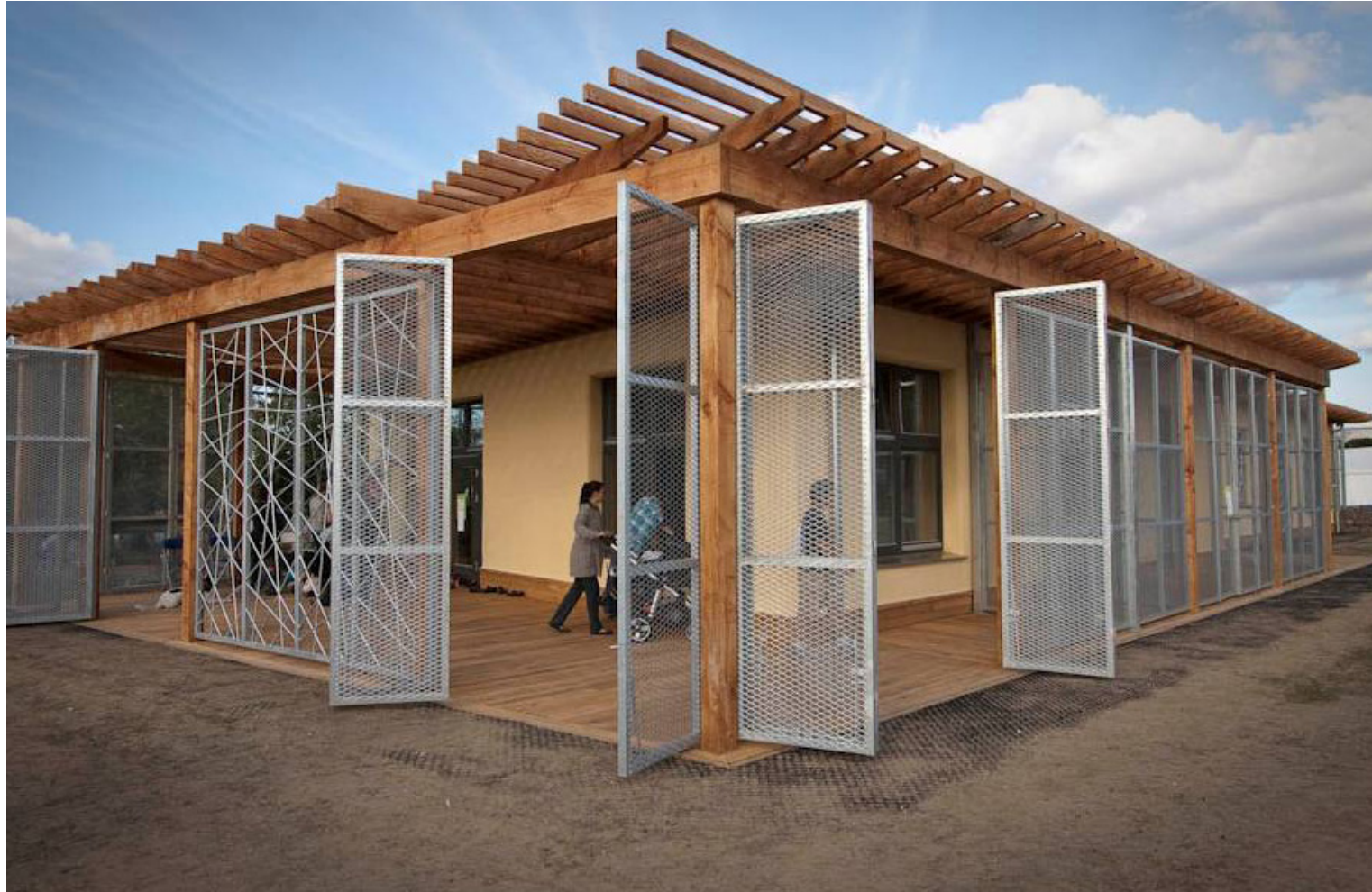
Figure 4: Passivhaus design, Lordship Recreation Centre, Haringey
