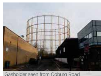
Gasholder seen from Coburg Road
