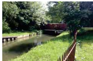
New River running under Station Road
