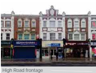
High Road frontage
