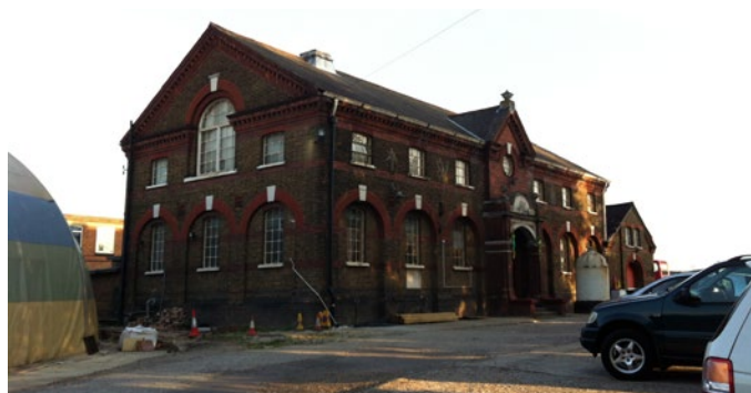
Historical Interest: The Marsh Lane Pumping Station in Tottenham is illustrative of an aspect of the area's history - the rapid development during the late Victorian era including important expansion of infrastructure.
