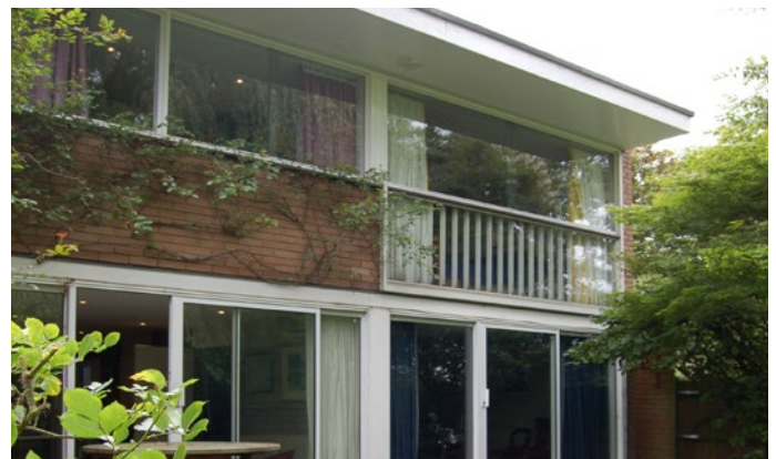
Innovative or Influential: This prefabricated house (below) and the small garden house (above) in Highgate were built by the architect Walter Segal as prototypes for his later prefabricated self-build houses including Segal Close in Lewisham.
