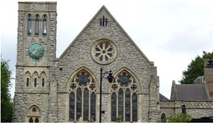
Architectural Interest: This former Presbyterian Church in Highgate is an attractive example of church architecture in the Victorian Gothic style.
