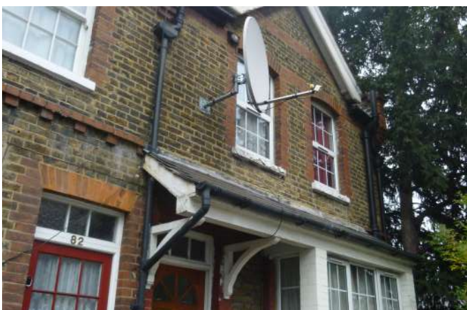
Satellite dish and replacement windows
