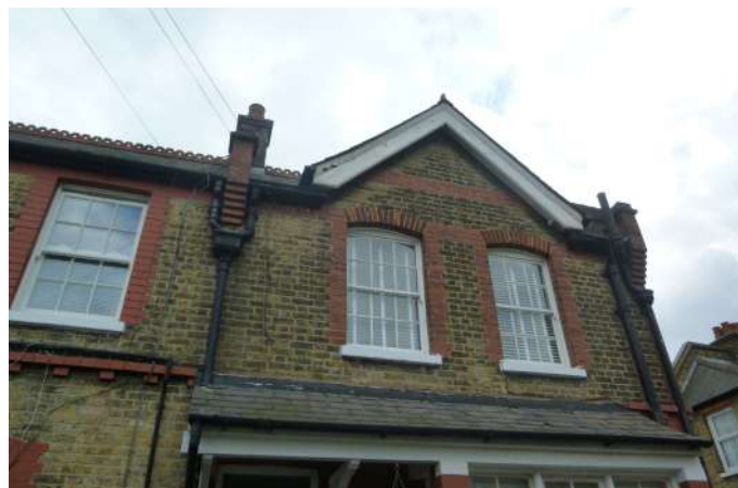
Detail of typical end-of terrace house
