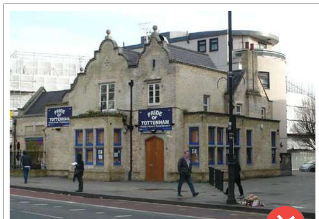
Extensions that are not subordinate to the original building can be detrimental to character
