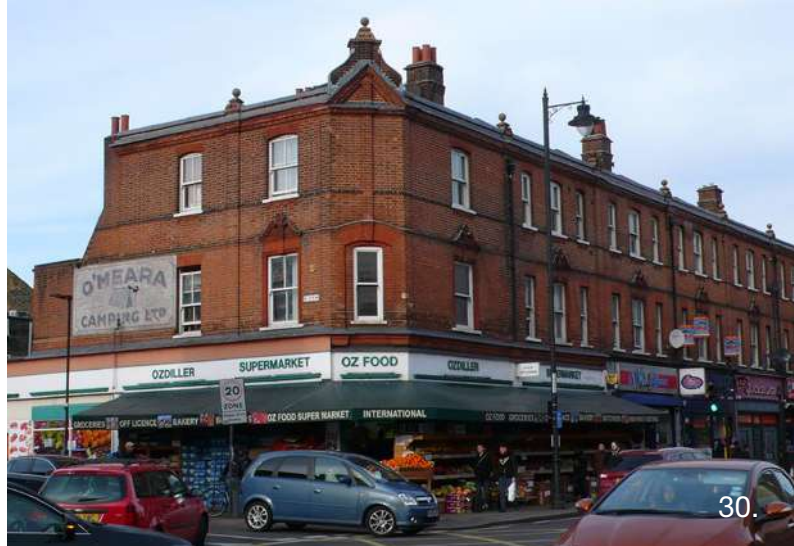
Picture 29. Mosaic Fascia at 479 and 481 High Road, compromising the appearance of Warner Terrace
