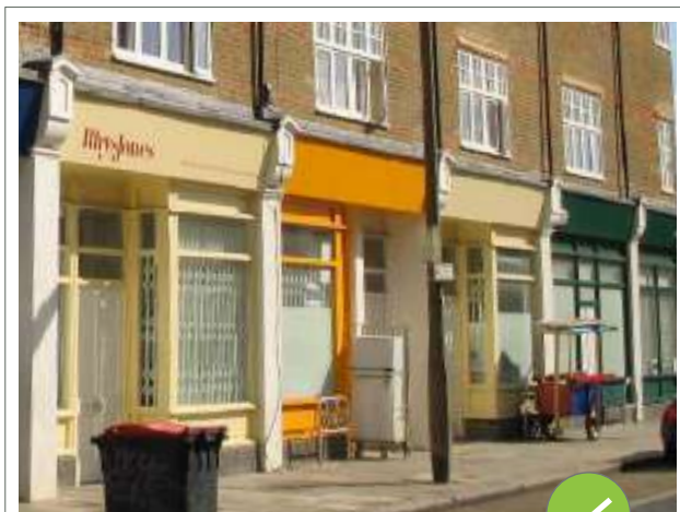
Internal shutters which don't obscure architectural features
