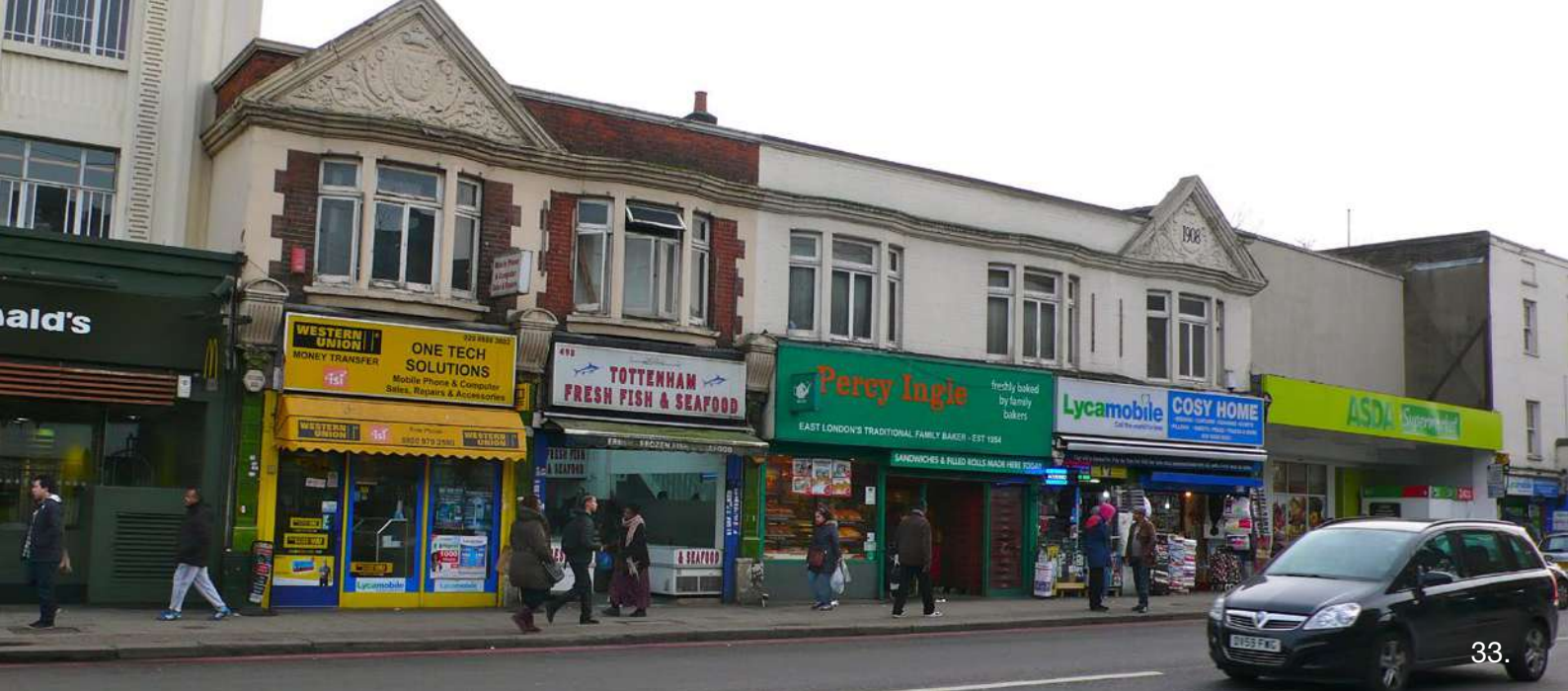
Picture 33. Two-storey parade at 492-500 High Road
