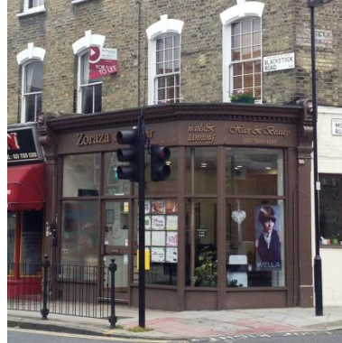
Photo 29: Locally listed building
