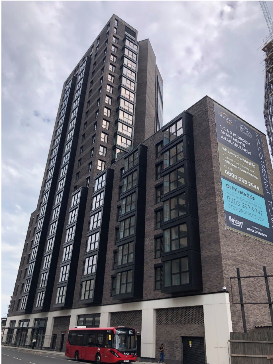
Image: Newlon Housing Trust, Millstream Tower – 117 Shared Ownership and 11 private sale homes.
