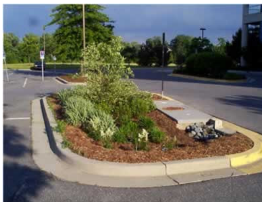
Figure 11 – Illustration of an engineered bio-retention area
