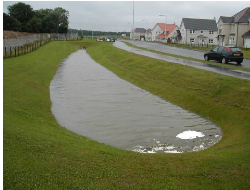
Figure 12 – Illustration of a detention basin following a period of heavy rain
