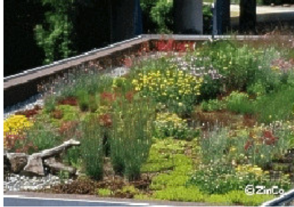
Figure 5 - Illustration of an extensive green roof
