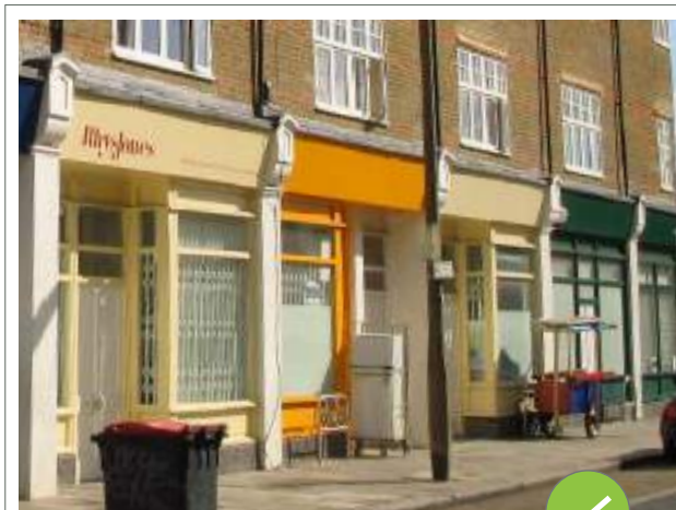
Internal shutters which don't obscure architectural features
