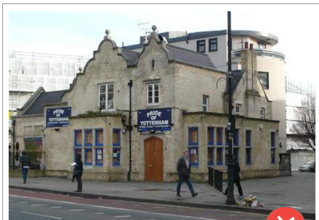
Extensions that are not subordinate to the original building can be detrimental to character
