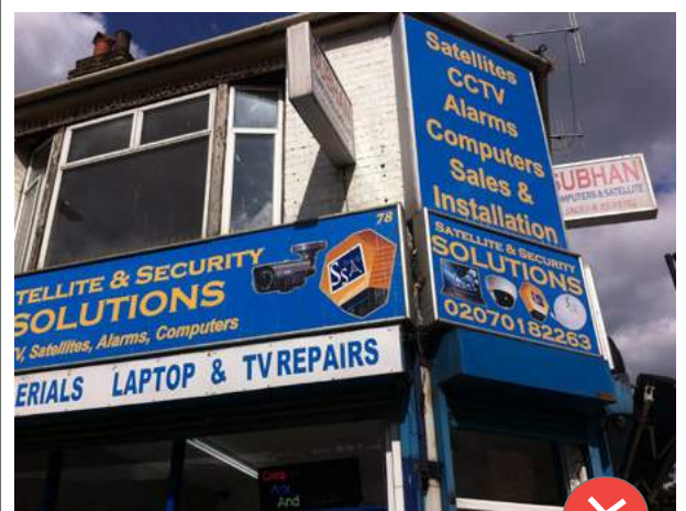
Windows should never be replaced with a different style or configuration to the original
