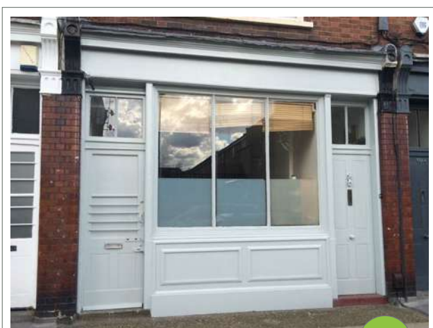
Original shop front features should usually be retained and adapted.
