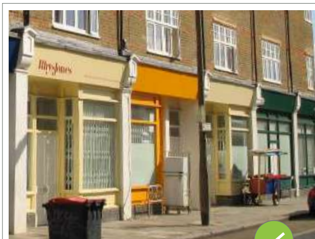
Internal shutters which don't obscure architectural features
