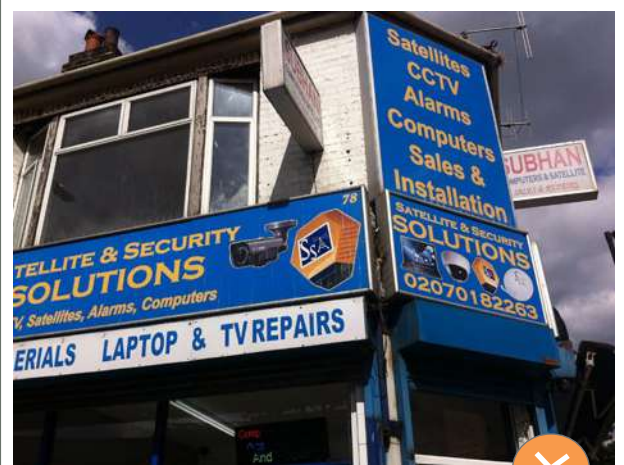
Windows should never be replaced with a different style or configuration to the original
