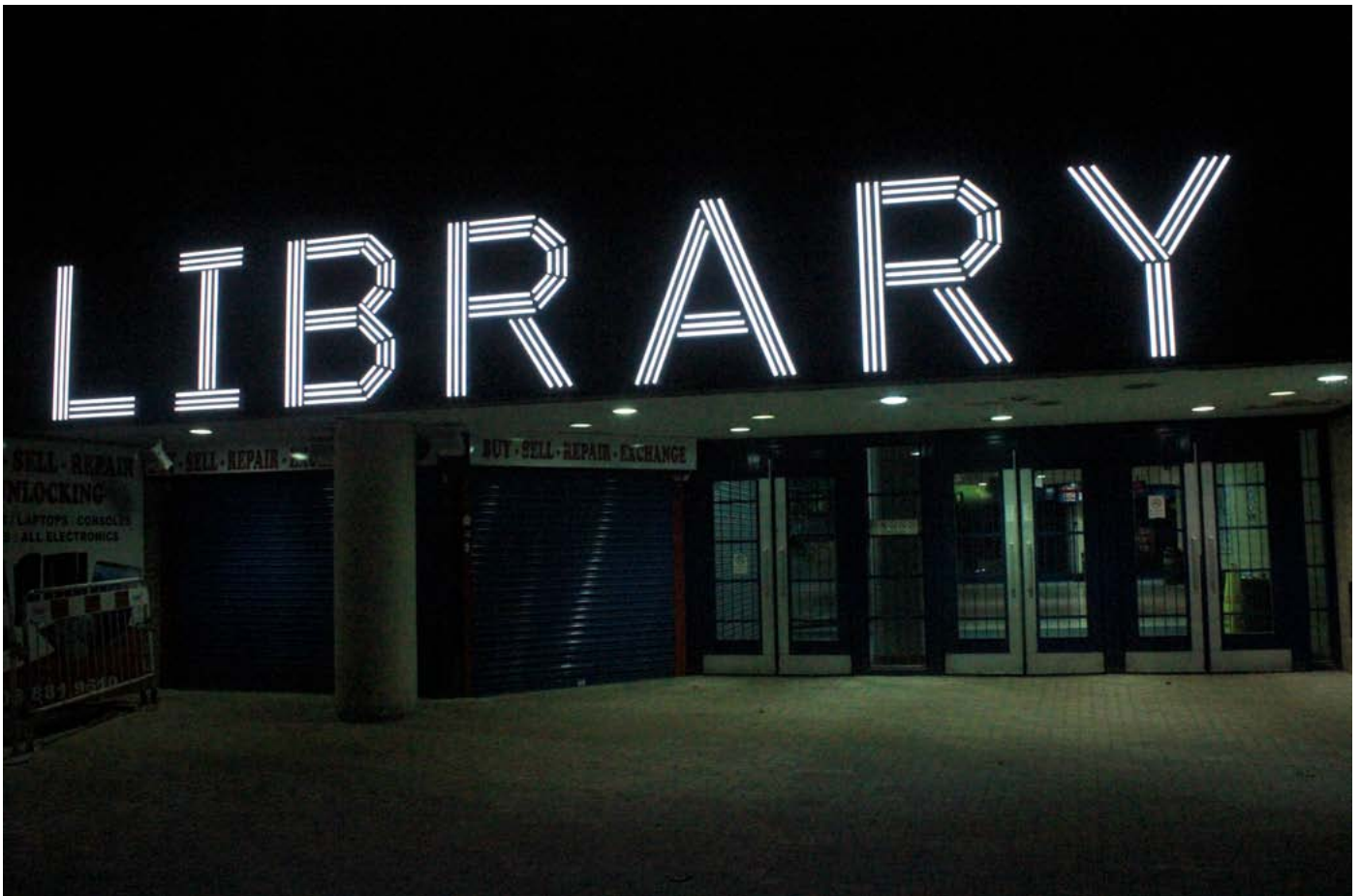
Despite recent public realm improvements the space in front of Wood Green library relies heavily on the illuminated 'Library' signage
