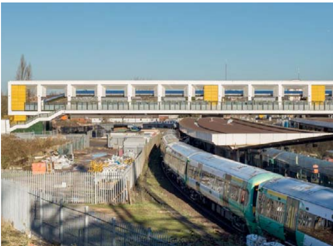
East Croydon Footbridge by Hawkins / Brown
